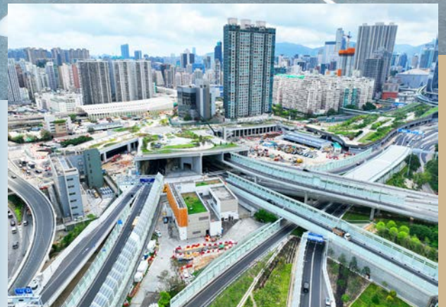
The western side of Central Kowloon Bypass (Yau Ma Tei Section) – Yau Ma Tei Portal
