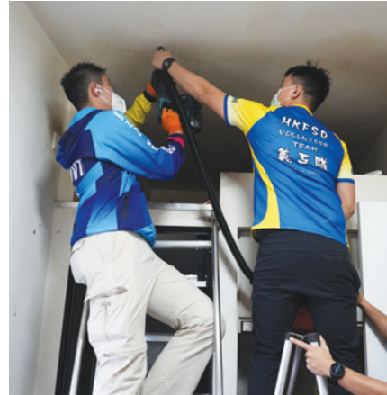
Installing stand-alone fire detectors.
