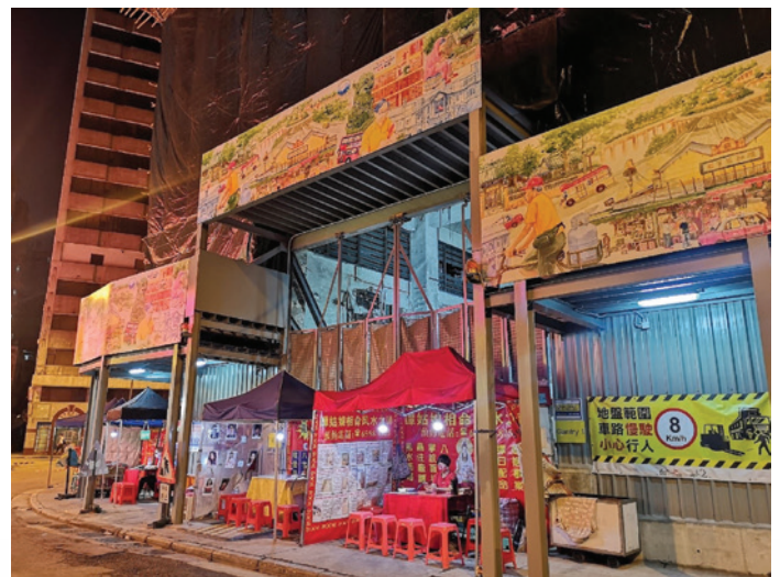
Unique design of temporary covered walkway suits the hawker stalls in the vicinity.
