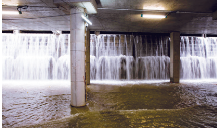
Happy Valley Underground Stormwater Storage Scheme.
