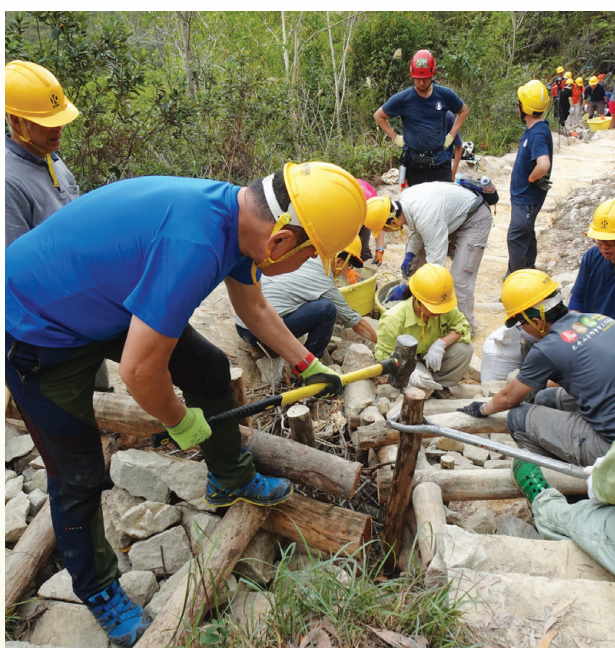
Trail volunteers work together on trail maintenance.
