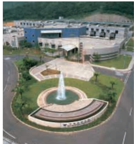
The Ngau Tam Mei Water Treatment Works is one of the most advanced treatment plants in the world.
