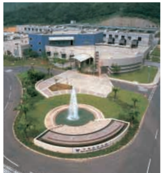
The Ngau Tam Mei Water Treatment Works is one of the most advanced treatment plants in the world.
